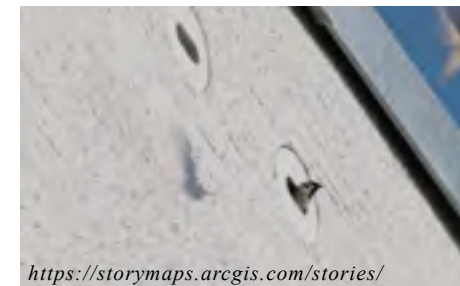
Innovative design of the facade of the building to provide house spawors with nesting alcoves (accessed 10.08.2023)
