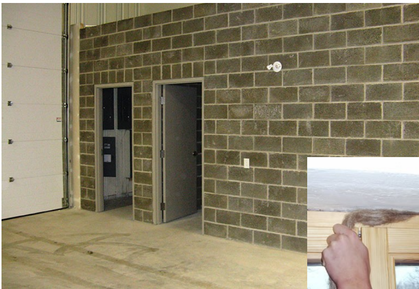
Figure 3: Wall constructed of Hempcrete – a biocomposite material consisting of hurd, lime, water and a binder.
